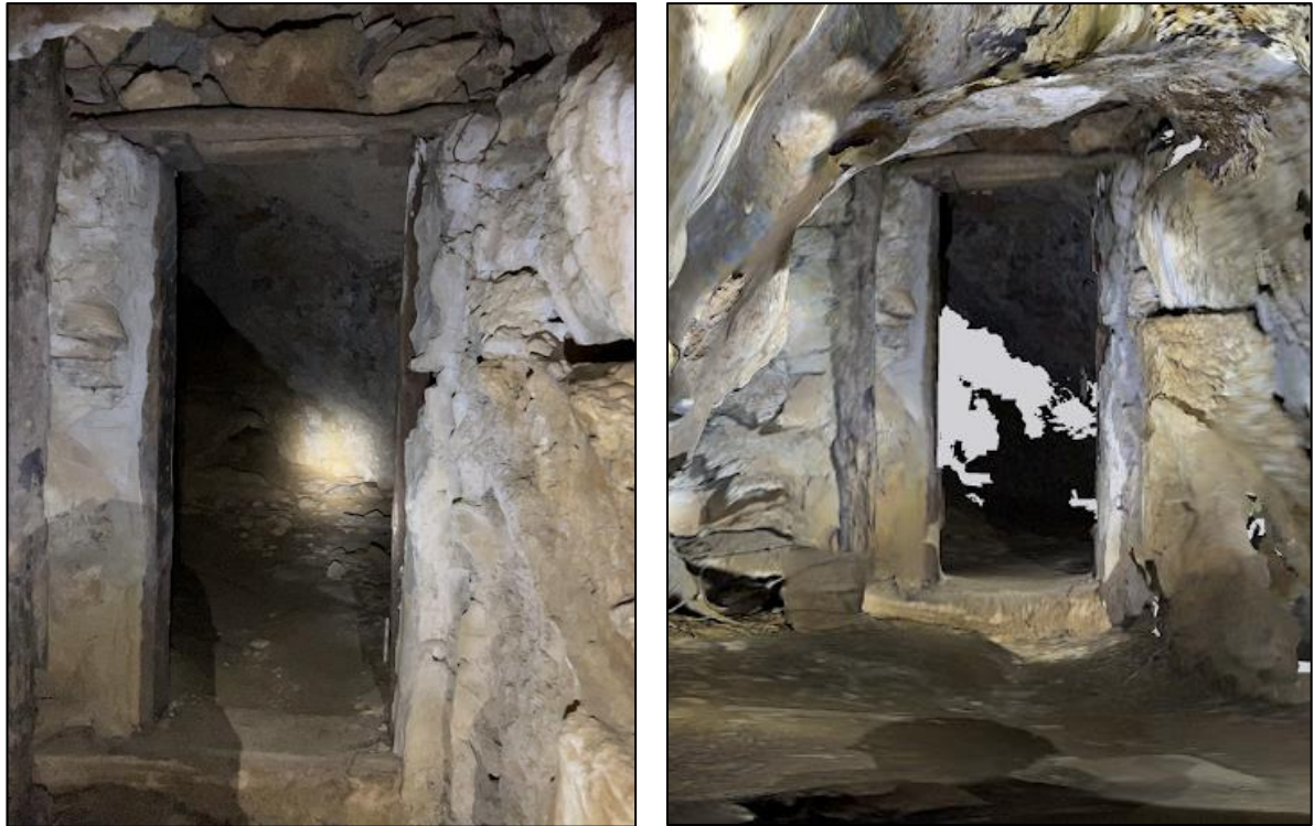
Figure 18. Door frame built in the Macumba cave. (Left) Picture captured with iPhone 13 Pro Max and the Scanner 3D App. (Left) Reconstruction of the doorframe.
