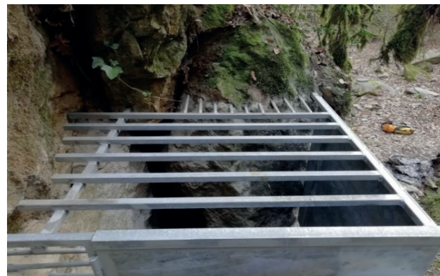
Figure 7: A cave protected with a door leaving a passage for bats. Photo: Christophe. Bes.
