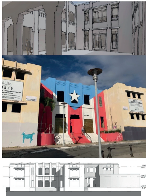
Figure 4 : This structure is the future home of the Instituto del Karso de Puerto Rico y el Caribe (Karst Institute of Puerto Rico and the Caribbean or IKPREC) (photo of building facade by M. Pérez, 2022).
